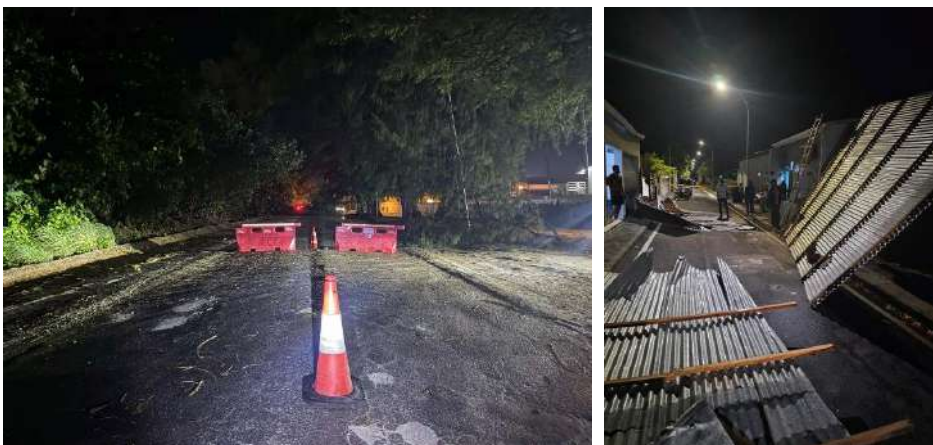
Figure 43: (left) Addu Link Road blockade due to fallen trees, (right) Roof damage in S. Maradhoo Feydhoo
